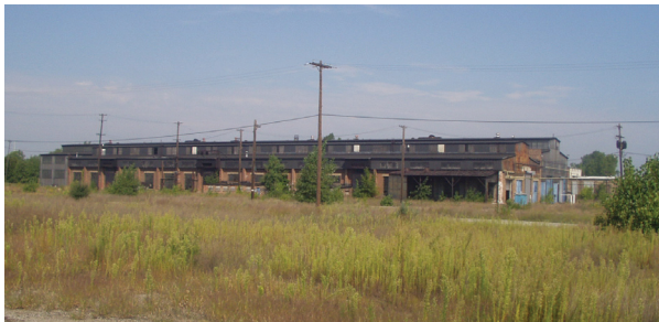
Abandoned rail car maintenance buildings south of Griswold Road and west of 28th Street
